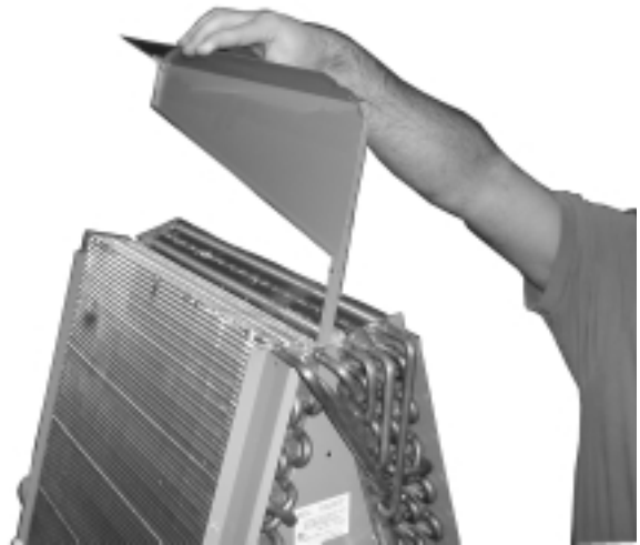
FIGURE 9 ROTATE DRAIN TROUGH
